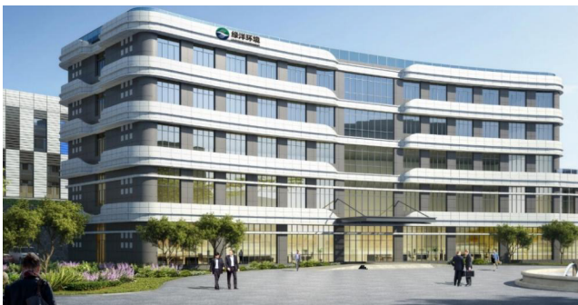
Figure 1. Leadyoung new office building (under construction)
